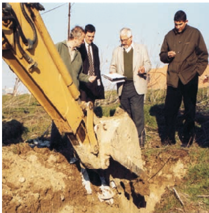
Subsurface geological exploration to acquire soil samples for laboratory analysis.
