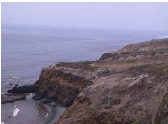
Coastal bluff landsliding poses a serious constraint at this potential site.
