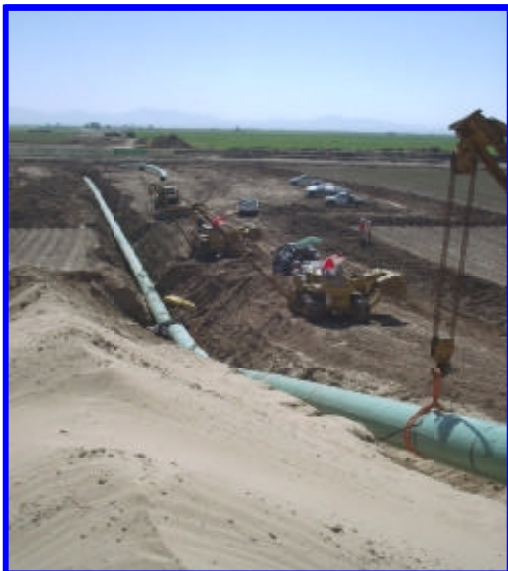
Pipeline Installation at the western margin of the Colorado River floodplain
