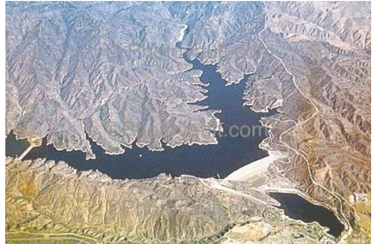
Aerial photograph of Castaic Dam in the San Gabriel Mountains. Photograph courtesy of Wernher Krutein.
