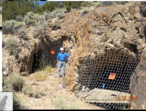
Mt. Hope is the site of the future General Moly molybdenum mine (left). The southern flank (shown) is proposed for mine infrastructure, but is undermined by old mine stopes (below).
